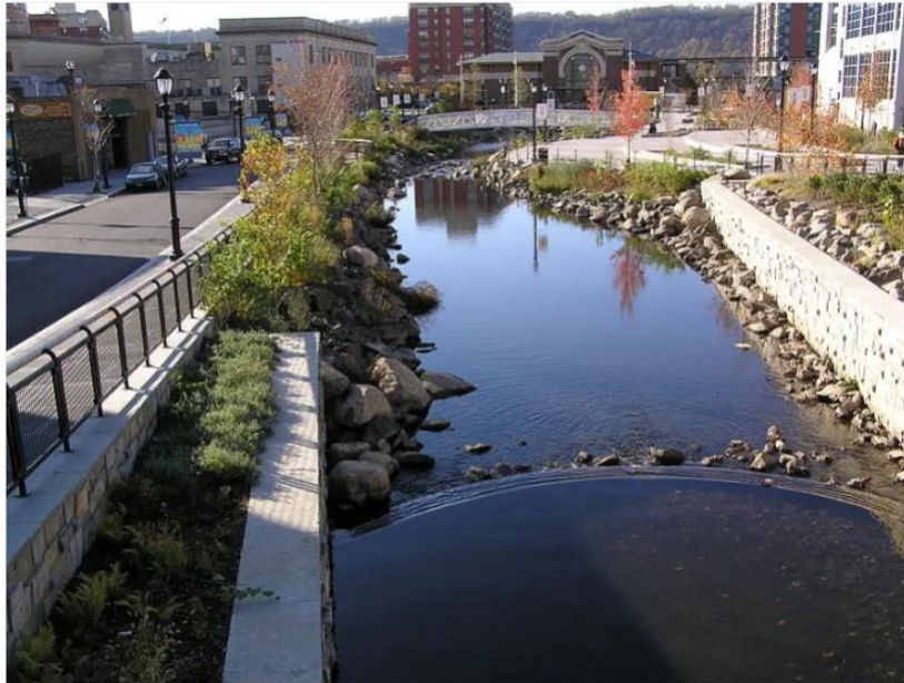
Buried underground for nearly a century, the Saw Mill River in Yonkers, NY in the USA has been daylighted in a $19 million programme, providing new habitat for a variety of life including the migratory American eel. Image: Wikipedia.
